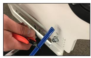
11. At both ends of the blue Flexirack, use two of the small metal clamps (see Parts List, item B) to hold the ends firmly in place. The clamps have a hole through the center and a lip on one end. The lip should be on the side opposite the blue Flexirack. Place the clamps where they will be attached and drill pilot holes using the 3/32-inch drill bit and then use a Phillips screwdriver to fasten the clamps on both sides of the Flexirack to the table.
