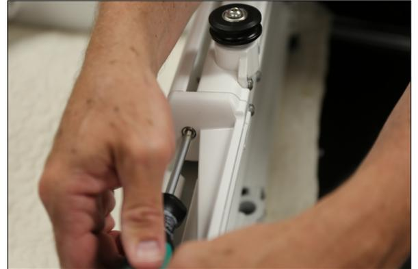
6. Then use a 5 mm hex tool to fully tighten the screw you loosened in step 1.
